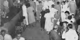
The large restaurant section easily held the several hundred guests at the reception that followed the dedication of Aruba's new airport building.
